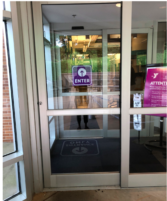
Figure 4. Automatic sliding door at entrance providing plenty of room for wider power chairs at your entrance.
